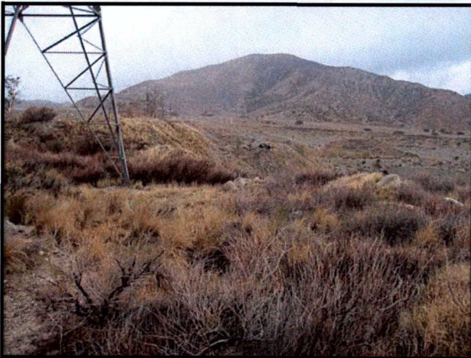
Photo 3: Devers-Vista #1 and #2 tower leg, adjacent to East Pit. Distance from the tower leg to the brow of a 100-foot-high descending cut slope (out of view) was measured at 17 feet. Foreground vegetation could be representative of "natural" conditions, as the tower footprint is one of the very few and very small areas of undisturbed ground.
