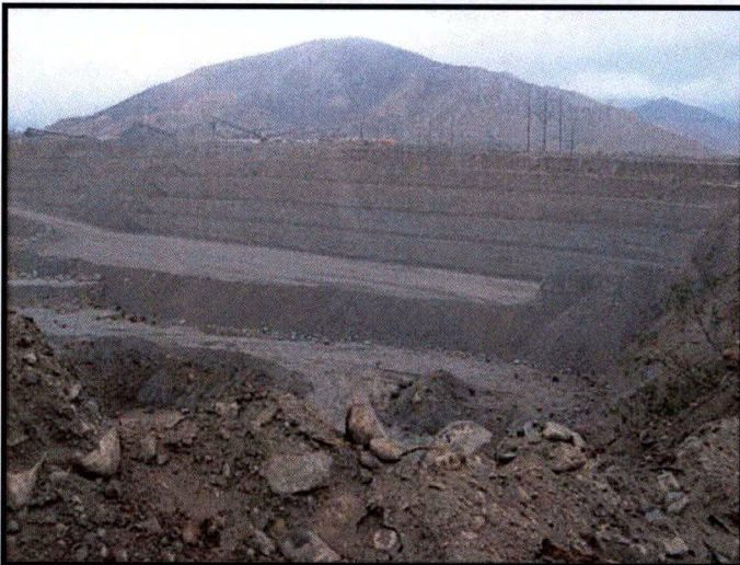
Photo 5: South Pit, view north. The northern pit wall has undergone slope trimming with a dozer and slope board, to create a benched surface with benches estimated at 20-foot intervals. The South Pit has been the primary aggregate source for the last year.
