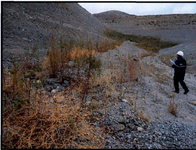
Photo 1: West pit, view north toward northwestern re-entrant corner. Engineered slope trimming has created smooth 1:1 bench face slopes with ~12-foot-wide benches. Since 2012, spring water inflows have almost completely ceased (former pebbly streambed in foreground is dry). Winter rainfall the previous season was near a historic low, however, and we expect surface flows in most years. No work has been done since previous inspection to control slope erosion or piping in the corner. Some floor areas of the West Pit appeared very recently mined, but inactive on the inspection date.
