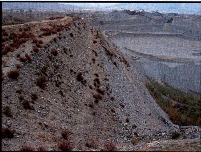
Photo 6: West Pit, view east along the northern highwall to show start of natural vegetation restoration. Noted that benches are becoming indistinct under a surficial cover of loose talus. Dense tamarisk is present where perennially saturated ground has been experienced due to spring flows (lower right). Pit bottom shows evidence for some extraction. Future resources continue east, under the existing plant site. The operator affirmed that relocation of the processing plant to the bottom of the South Pit is planned and will be documented in a new site-wide Reclamation Plan.
