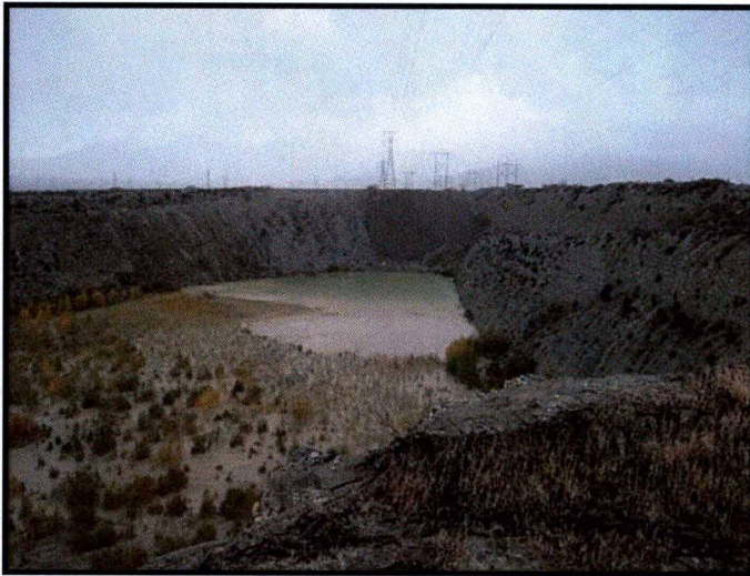
Photo 4: East Pit, view south from SCE easement. The eastern pit wall (left side) features loose soil slopes at natural angles of repose with some steeper projections of intact alluvial strata. The eastern slope approaches, but does not appear to cross, the property boundary with the adjacent Morongo Indian Reservation. This pit has been used for years as the disposal site for washed fines generated from the sand and gravel processing plant. Interpretations of CUP 1965 reclamation plans and the latest-available contour maps indicate that at least 17 feet of sediment is beneath the pond, thickening to the north. The \frac{3}{4} :1 cut slope in the right half of the picture has stood for at least 30 years. It has experienced some deep rilling and exhibits relatively sparse vegetation. It is believed this slope will be mined to pond elevation. Pondered water evaporates, or infiltrates into the excavation sidewalls.
