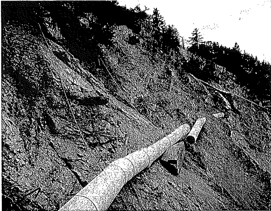
Figure 1: Temporary pipe in landslide area, damaged, looking downstream.
