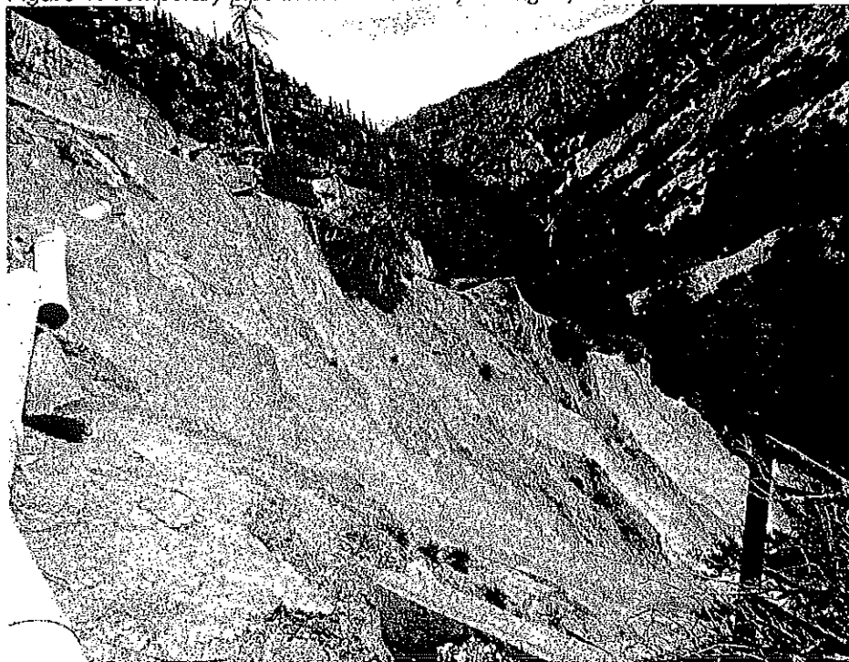
Figure 2: Landslide area, damaged flume, and damaged temporary pipe.
