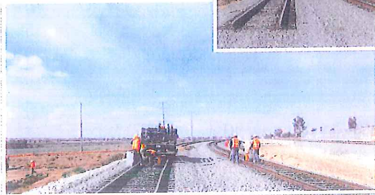
Removal of railroad "shoofly" tracks east and west
