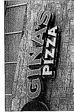
Creative use of cabinets with pushed through copy and dimensional icons are occasionally an excellent solution, when architecturally channel letters cannot be used.
