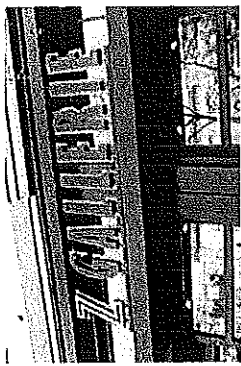
Individual internally illuminated channel letters mounted on canopy.
