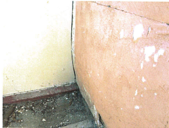
Buckled exterior plaster (rear)
