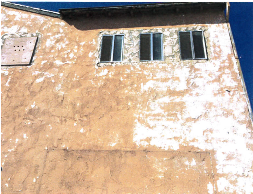
Deteriorating exterior plaster
