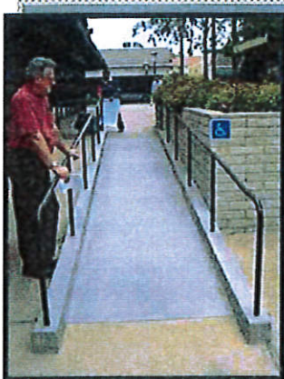
Redland City Hall ADA Renovation – New ramps and handrails
