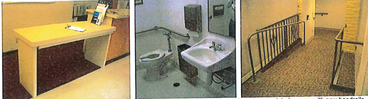
New ADA Compliance improvements at the Civic Center entry reception counter, public restrooms, interior ramp with new handrails
