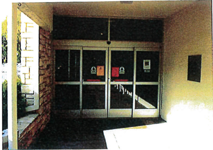
AFTER NEW AUTOMATIC SLIDING DOOR FOR EASY ACCESS TO COMMUNITY CENTER
