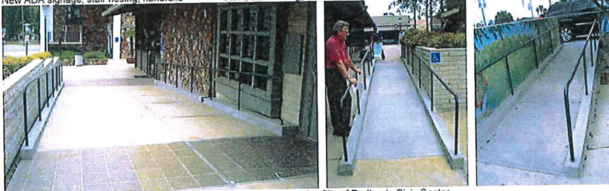
New ADA Compliant ramps, handrails, and ADA signage throughout the City of Redlands Civic Center
