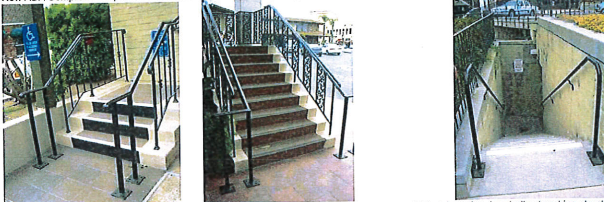
New ADA signage, stair nosing, handrails
