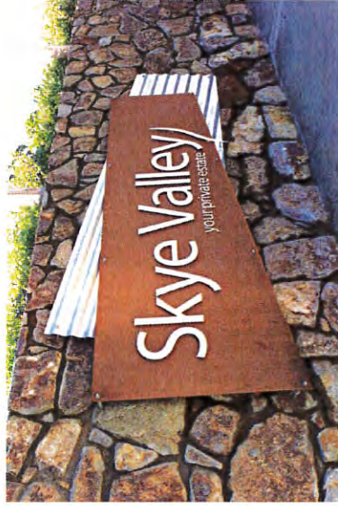
STAINLESS STEEL LETTERS ON COTREN STEEL PLATE
