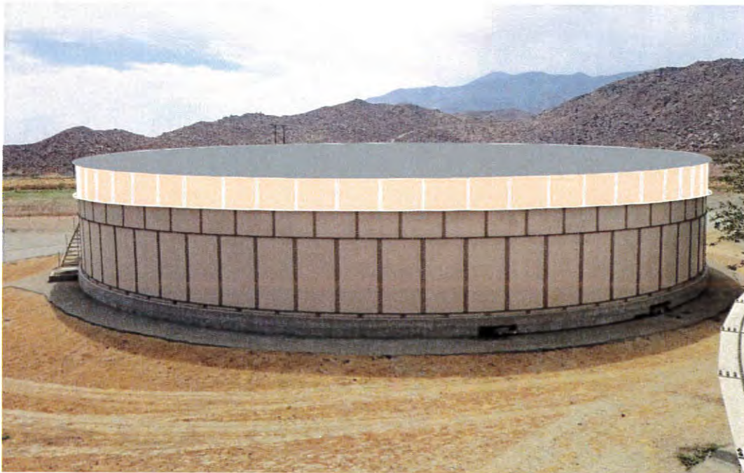
Figure 12: Profile of Added Ring to Increase the Volume and Height of Existing Trickling Filter
