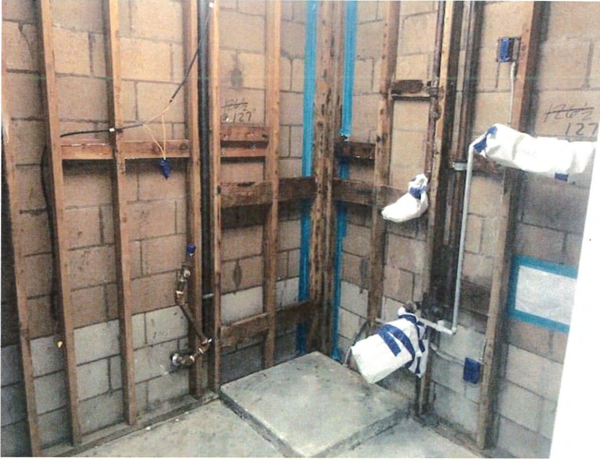
Figure 6: View from utility room. Water heater and affected drywall have been removed.
