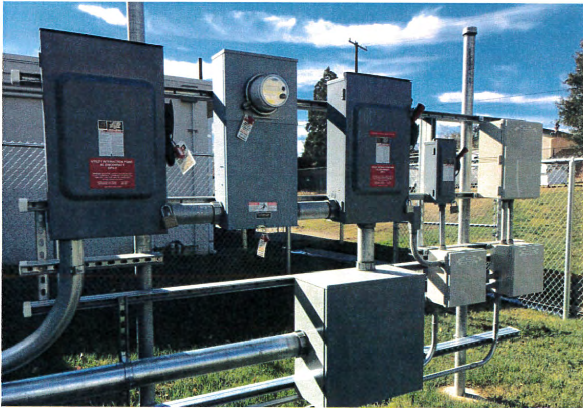
Solar PV Gross Meter, AC Disconnects and other components
