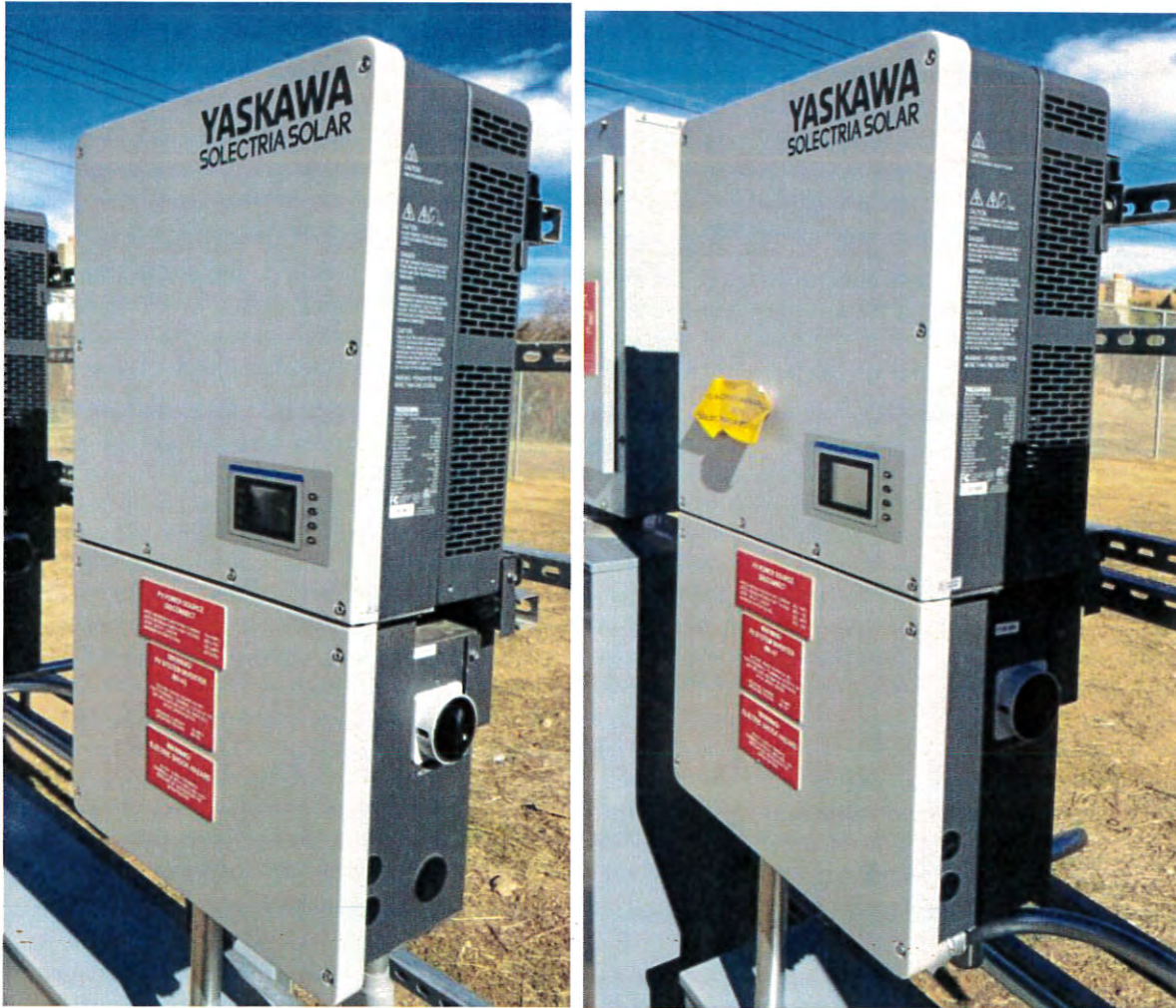
Two Solar PV Inverters
