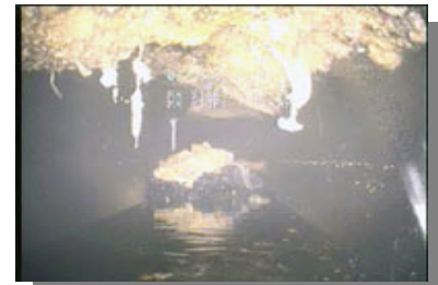
Figure 7-5 Grease Buildup – Sewer Main
