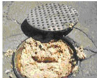
Figure 7-2 Plugged Interceptor
