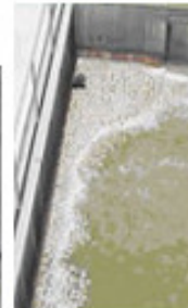
Figure 7-2 Plugged Interceptor
